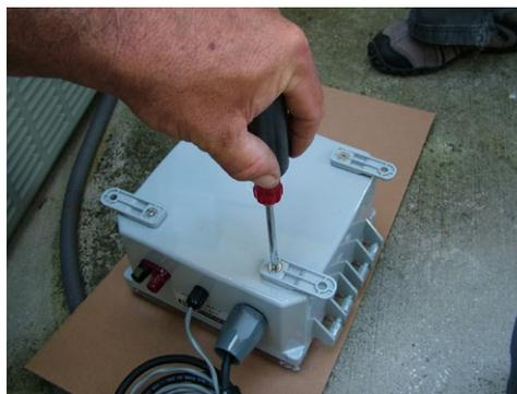
2.) Mount the microprocessor control box to the wall allowing for the power cable wire to reach the source of power; the electrode wire to reach the electrodes; and the **ScaleBlaster** signal cable to wrap around the pipe - also on the return line. Use proper anchors and screws to mount on the surface (wood, stucco etc.).
